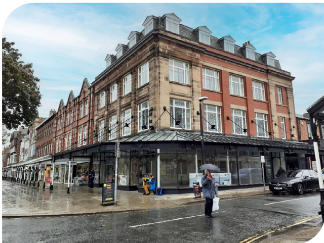
509-515 Lord Street, Southport: 2 vacant retail units able to be brought into use and vacant upper floors converted into 9 apartments.
