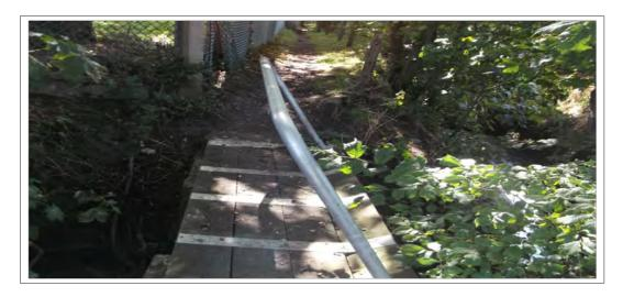
Image 15 Damaged handrail Melling footpath No. 11, report to **Structures, Development and Design.**
