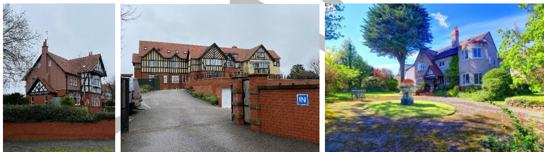
From left to right, No 42 Hesketh Road, No 40 Hesketh Road, No 21 Hesketh Road
