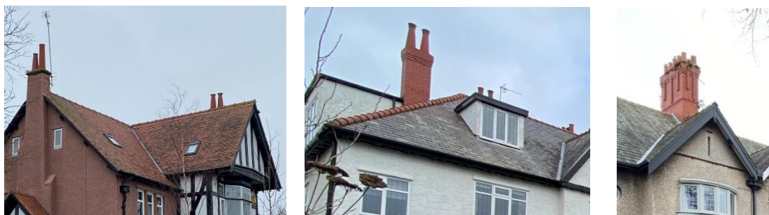
From left to right, example of rooflights and antenna, example of dormers, example of decorative chimney with some biological growth.
