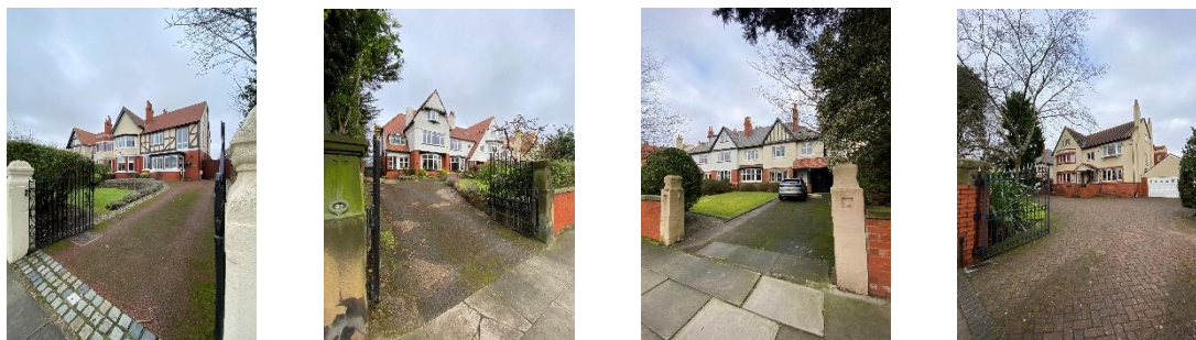
From left to right, Nos. 36, 32, 24 and 22 Hesketh Road showing the brick base at ground floor levels.
