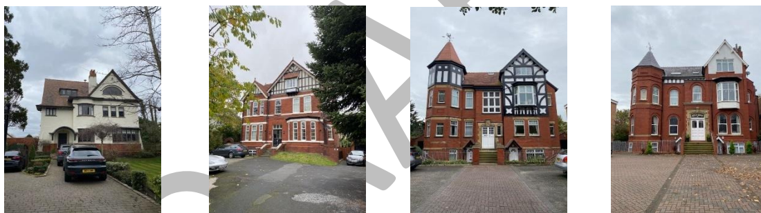
From left to right; No.28, No.27, No.18 and No. 14 (Holy Bank) Cambridge Road.
