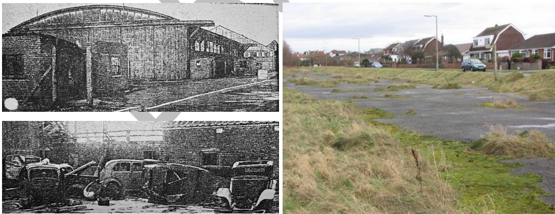
Photograph of the hangars in 1965 used to damp old cars. Remains of the apron are still visible today on site.
