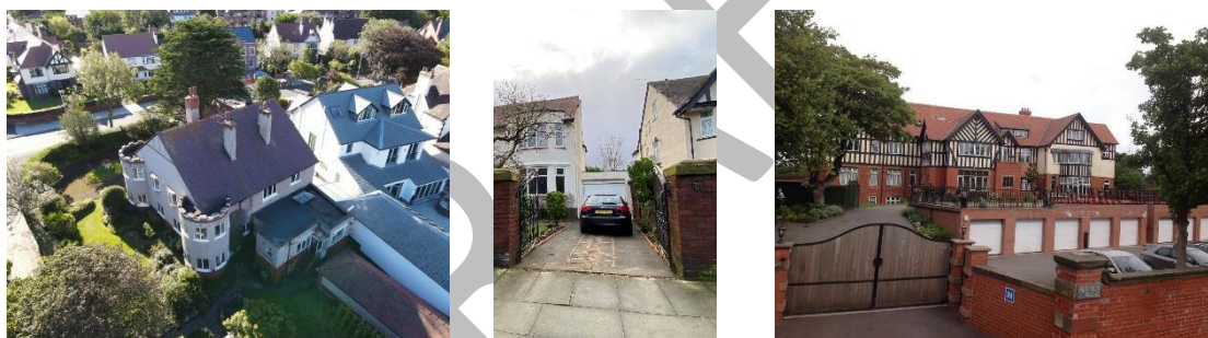
Examples of unsympathetic flat roof extensions.
