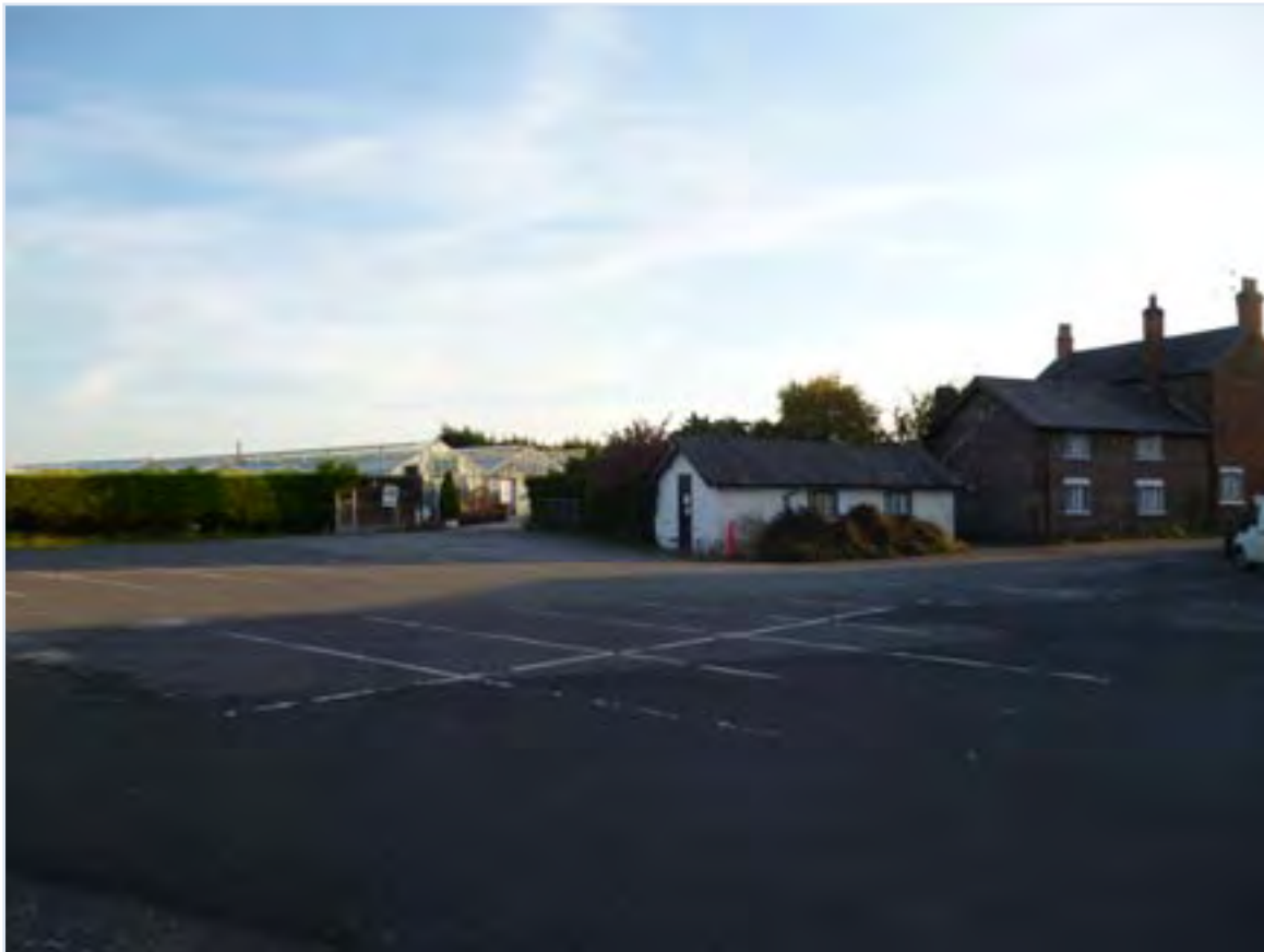
Plate AS 10- 3- Southeast facing view across the farmyard to the rear of Tan House Farm
