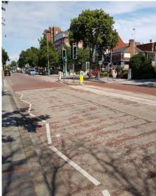
Large sections of the highway have become a patchwork of contrasting colours. Original stone kerbs can be seen within the Conservation Area, as well as modern concrete replacements
