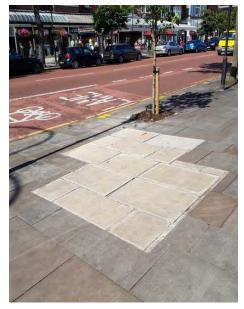
The tiles located outside of The Atkinson and the facing Civic Gardens are limestone, with sit alongside pre-cast flags. However, some are failing due to traffic here. More recent repaving works elsewhere within the central portion of Lord Street has replaced poor quality paving with a mixture of Indian sandstone and standard grey concrete flags. Tactile paving here has been more sensitively incorporated using similar stone.
