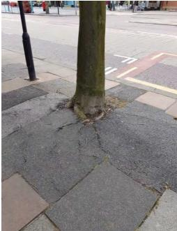
Some trees have been inappropriately covered in asphalt up to the trunk
