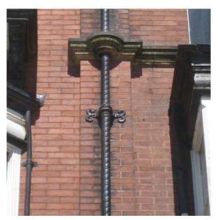
Cast iron 'rope twist' style downpipe and decorative brackets at 447-449 Lord Street, integral to design of façade.
