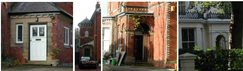
Porches within the conservation areas
