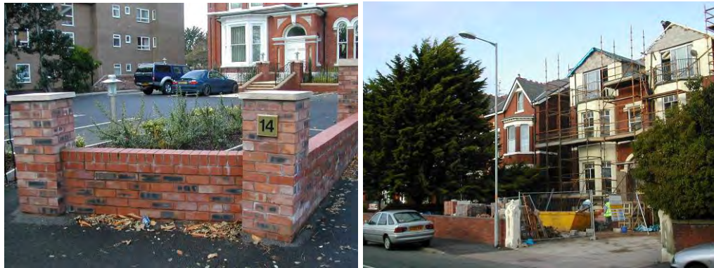
Replaced or lost gate posts and front boundary walls. The left-hand photograph also illustrates the loss of the front garden of the old villa to car parking.
