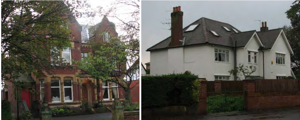
Examples of detrimental replacement windows and rooflights.
