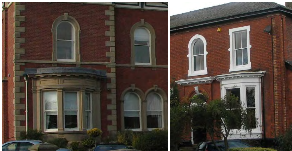
Sash windows within Birkdale Park
