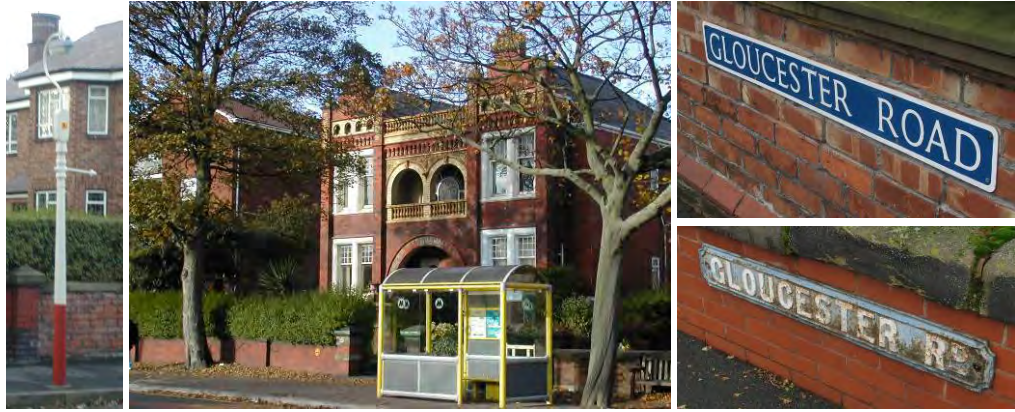
(Left) Older, converted lamppost; (middle) modern bus stop that adversely affects the setting of a listed building; (right below) early cast iron sign; (right above) modern replica sign that although uses the original colour scheme of the old street signage, is not of the same quality.
