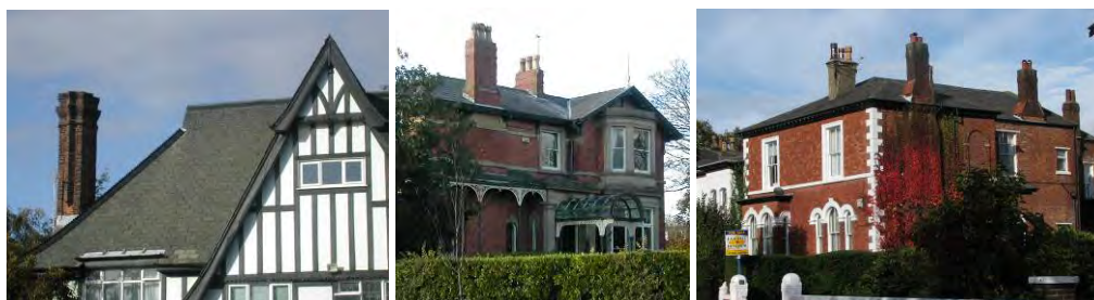
Chimneys within the conservation areas
